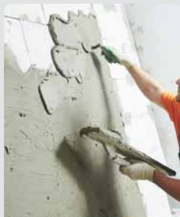
Internal plastering of walls & ceilings
